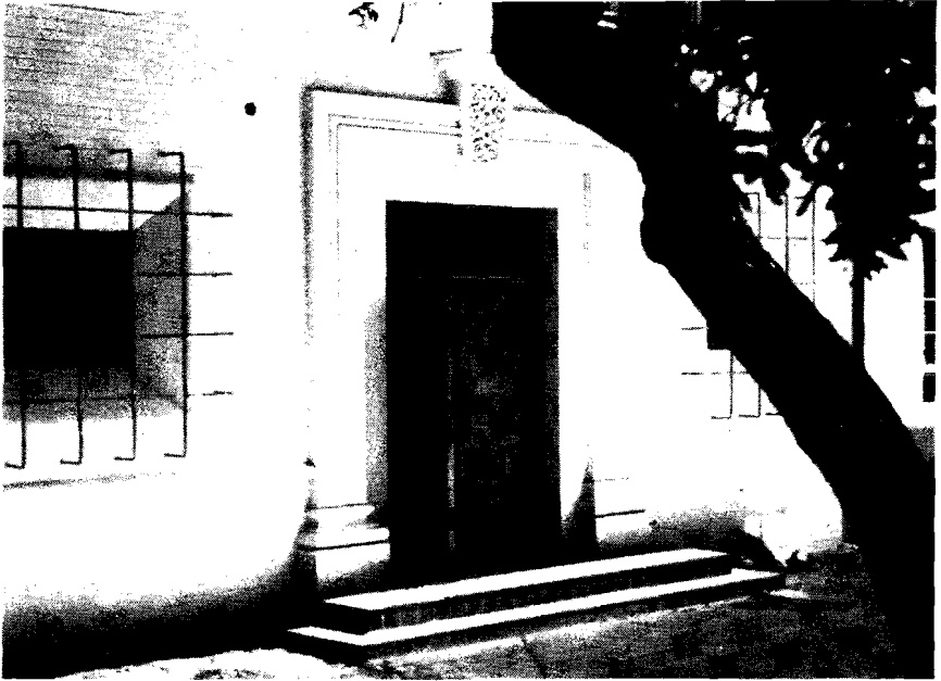
Fine Arts Doorway (Before Completion)
