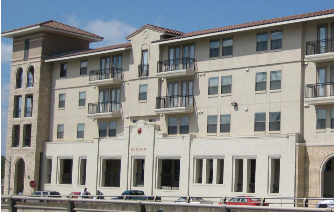
Figure 4: New structure at 300 N Lamar, offered as comparison of preservation technique
