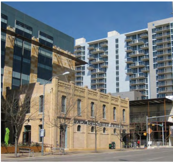
Figure 1: Schneider Brothers Building, Southeast view, February 28, 2008
