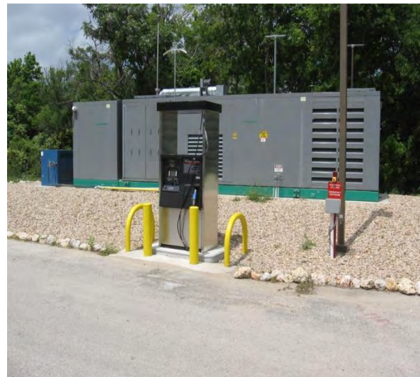
Image 2.5: This Hydrogen fuel station operated by the University of Texas was difficult to find. UT operates a hydrogen fuel cell bus.
