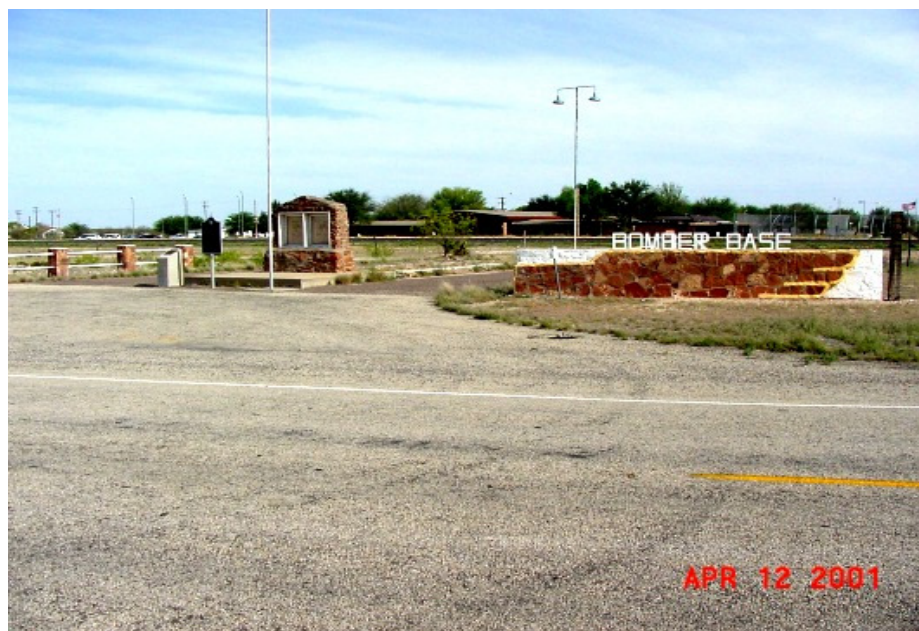
Figure B10. Restored front gate to Pyote AAF. 10
