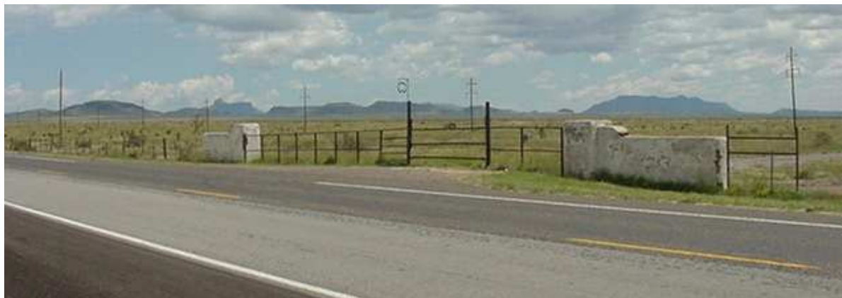
Figure B5. The front gates of Marfa AAF as they appear today. 5
