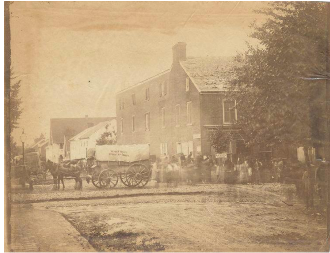
Figure 6.13: United States Sanitary Commission Branch, Gettysburg, Pennsylvania. 37
