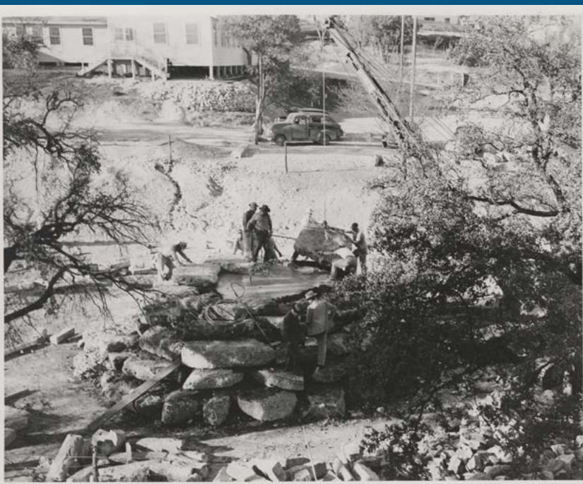
Constructing base for Fighting Stallions, circa 1952
