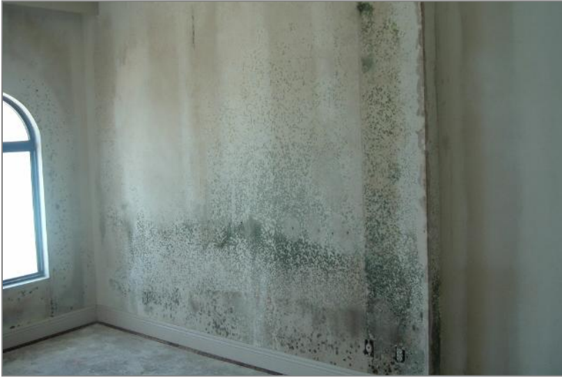
Mold on the Walls of Room 528 (left) and Pile of Carpets to be Discarded (right)
