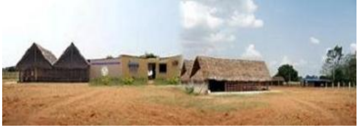
Figure 4. Shed of Britto Community College. A picture of the shed where Britto Community College was established in 2008.
