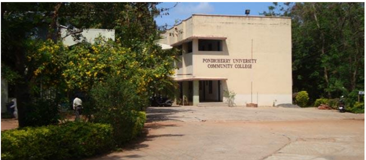
Figure 3. Pondicherry University Community College. Main Building of the College.
