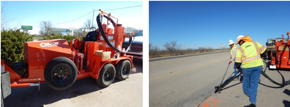
Figure 2-5. Hot pour crack sealant tank and its application
