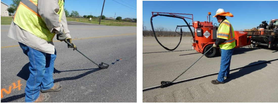
Figure 2-3. Squeegee for sealant
