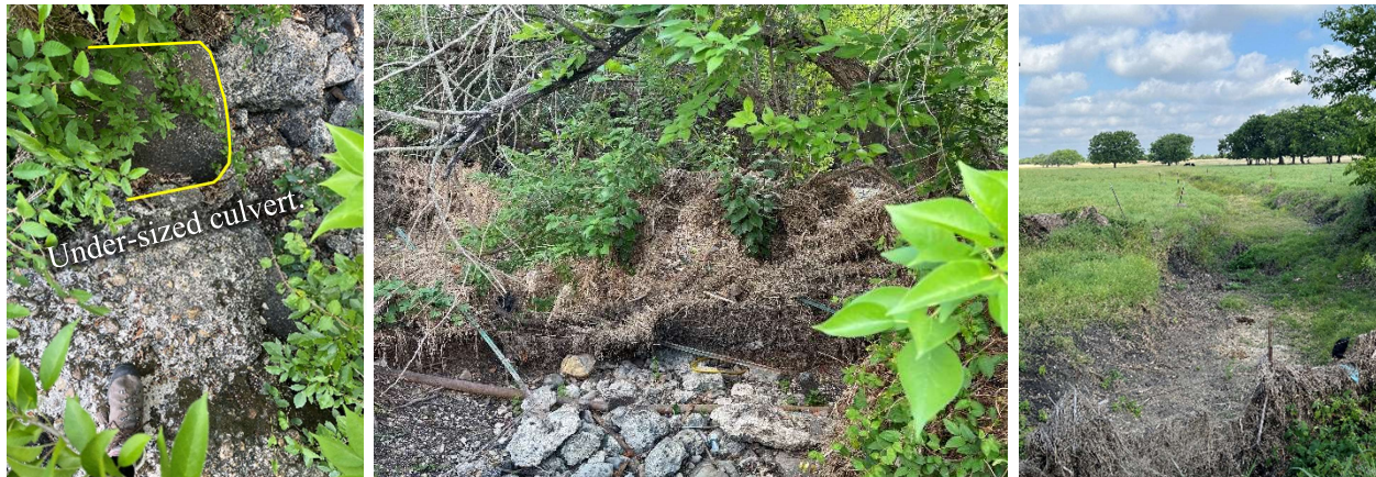
Figure 4. Under-sized culvert, debris caught in fence, and chute cut-off leading to off-channel pool at crossing at Stueve Lane.
