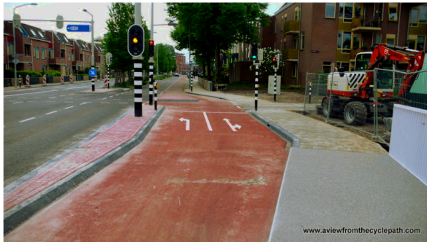
Figure 5 - A typical Dutch shared use street. The cycle path is visually distinct from the roadway. Note especially the intersection, where the bike lane is separated further from traffic by a concrete curb and dedicated traffic-signal device. This particular cycle path is one of the newest (as of May 31, 2016) cycle facilities in the Dutch city of Assen, and is cited by David Hembrow as an example of improved design in cycling facilities for widening at a potential bottleneck. Photo Credit: David Hembrow, A View From the Cycle Path Blog , retrieved on June 15, 2016 ( http://www.aviewfromthecyclepath.com/ )
