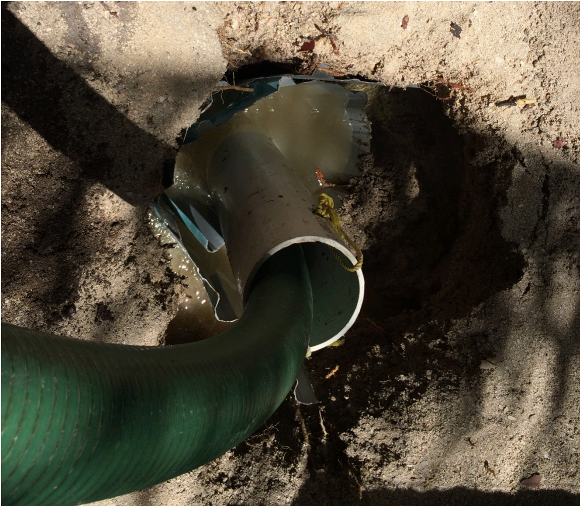
Figure 16. Pump intake hose with sheet metal support
