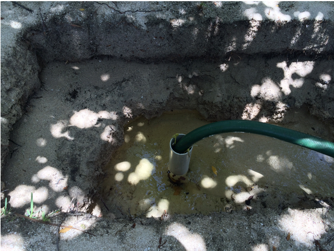
Figure 15. Pump intake hose with the vertical synthetic pipe
