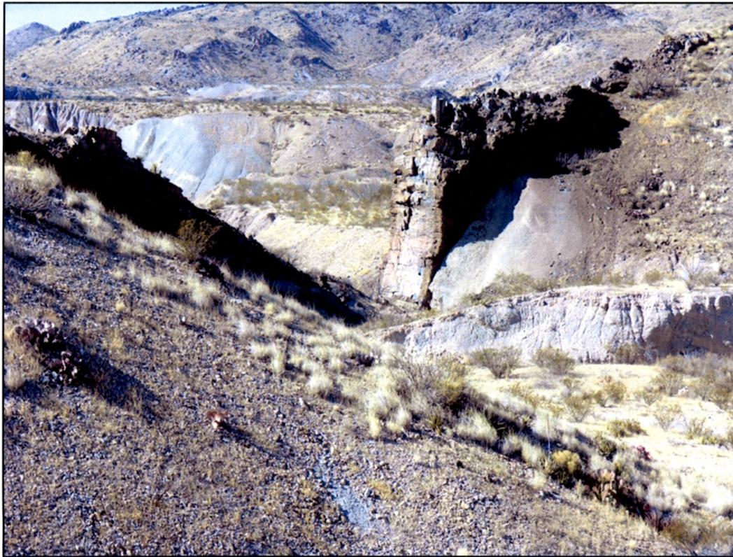
Figure 2. Downstream view of a breach in the dike.
