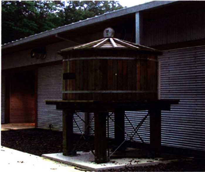
Figure 2: Seven hundred gallon rain cistern for storing rainwater for the Camp Aldersgate Commons Building, Little Rock, Arkansas (Source: Mark Littrell, Wilcox Group Architects)
