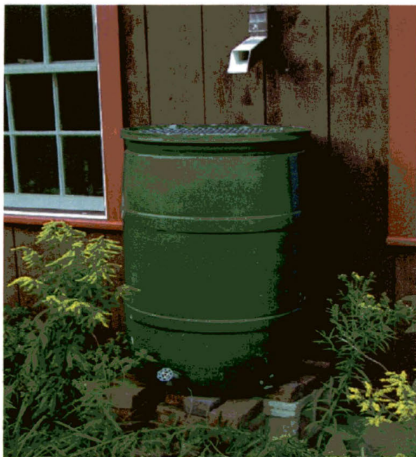
Figure 3: A rain barrel, including spigot and connection to downspout (Source: Lake Co. Illinois Stormwater Management Commission)
