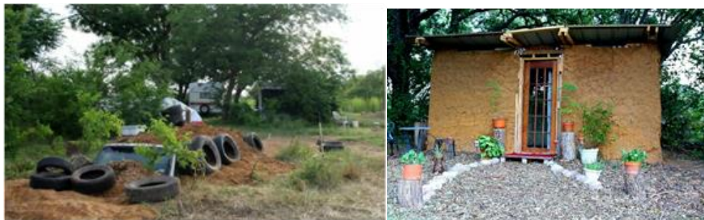
Figure 6: Buried Vehicle. A partially buried vehicle with tires and vegetation as insulation, a model of sustainable housing. Figure 7: Sustainable housing. Pictured on right is a small cob cottage with a salvaged door. Images obtained with permission from The Garden of Eden ( http://www.intothegardenofeden.com ).
