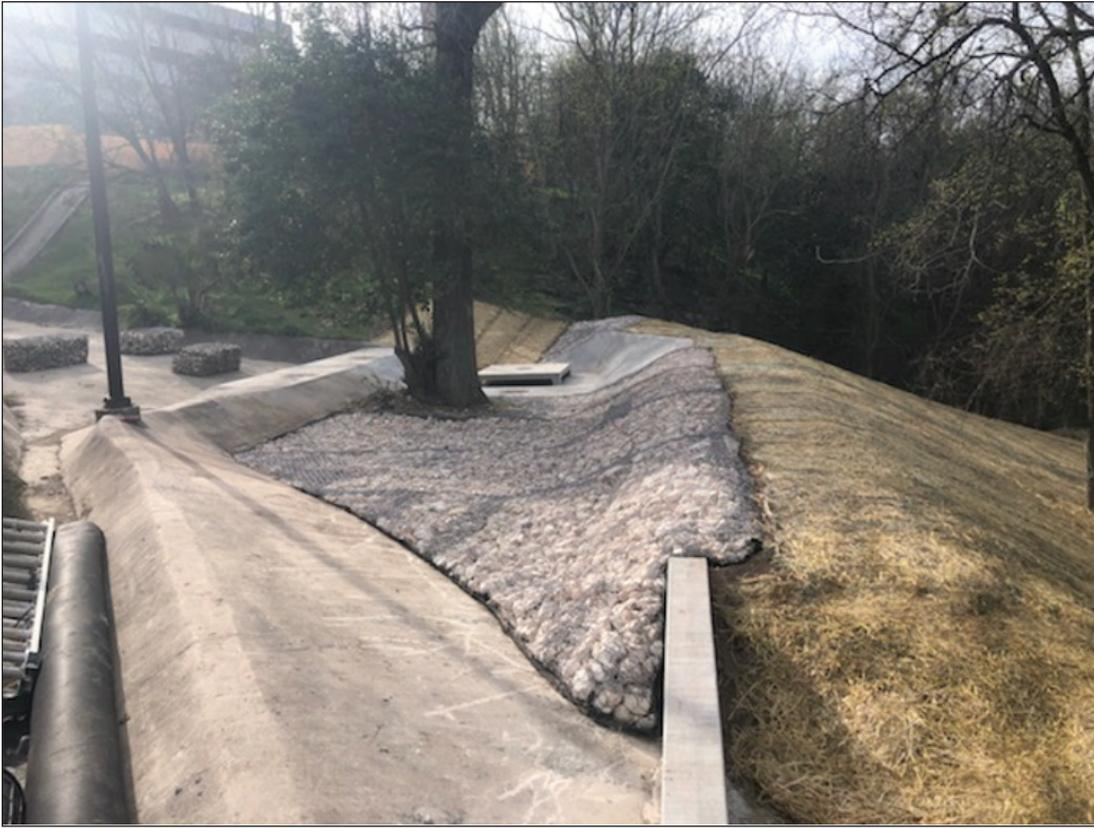
**Figure 3.** The completed Hogtrap Retrofit, showing the inlet before the piping goes below the surface. (Photo courtesy of Joey Kristoff)
