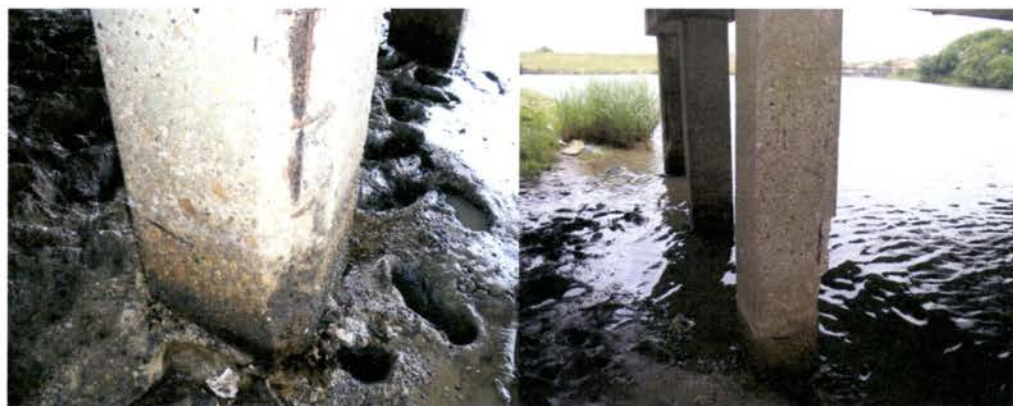
Figure 4: Overview of the level of deterioration at SH 82 at Alligator Bayou (Jefferson County)
