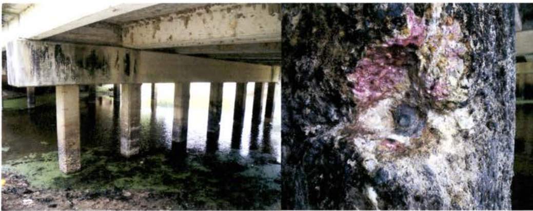
Figure 5: Overview of the level of deterioration of SH 31 West Bound at Kickapoo Creek (Henderson County)
