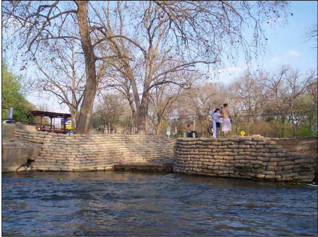
Illustration 26. Site 11: Sandbag Retention Wall, March 2006. Source: author.
