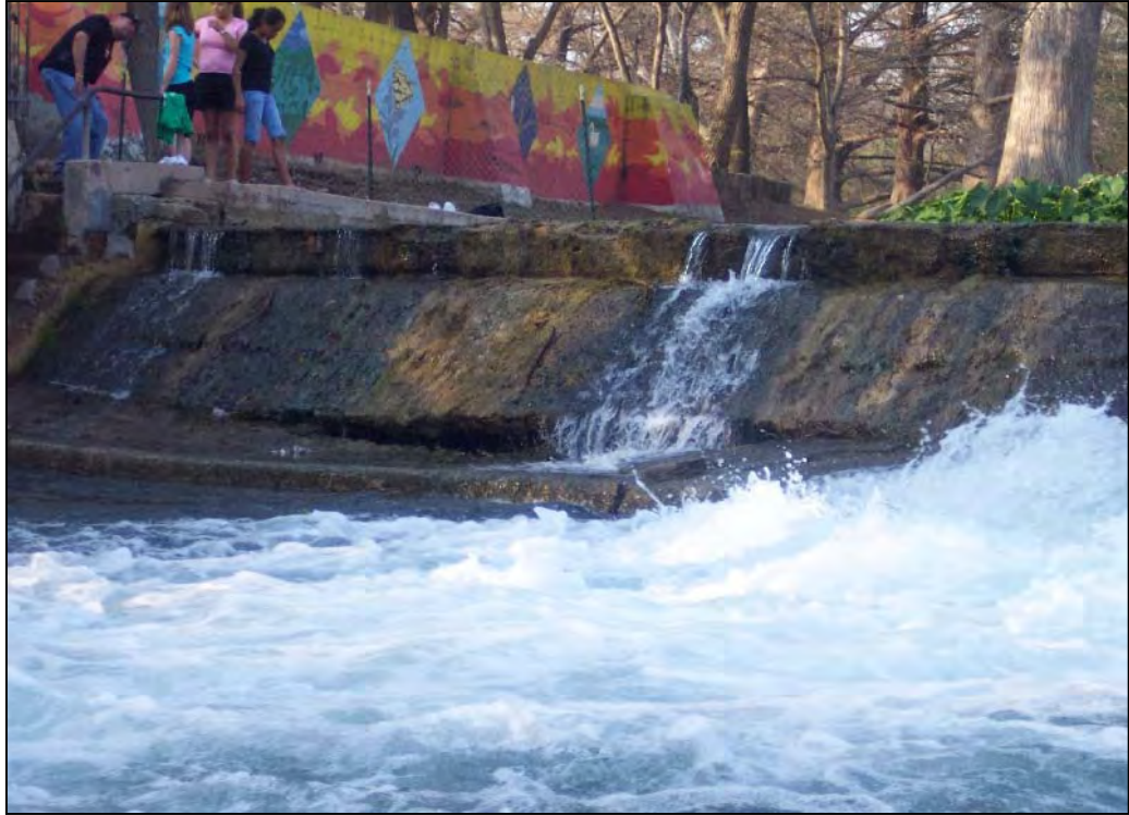
Illustration 24. Site 10: Close-up of Break in Dam, March 2006. Source: author.
