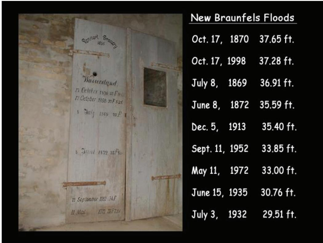
**Fig. 4.** Documented flood peak marks on the door of old brewery located on the bank of the Guadalupe River in New Braunfels, Texas.
